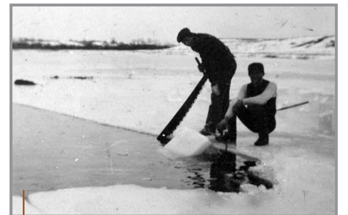
Cutting ice in 1911, on Spring Lake on the south end of the Maybee farm. Ice was stored for year-round use before electrical refrigeration became common.
